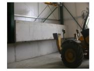
Panels are fixed to the stanchions using the plates and bolts provided.
